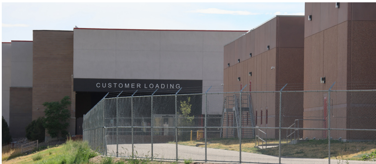
Exterior of the GEO facility in Aurora, Colorado, August 2024.
